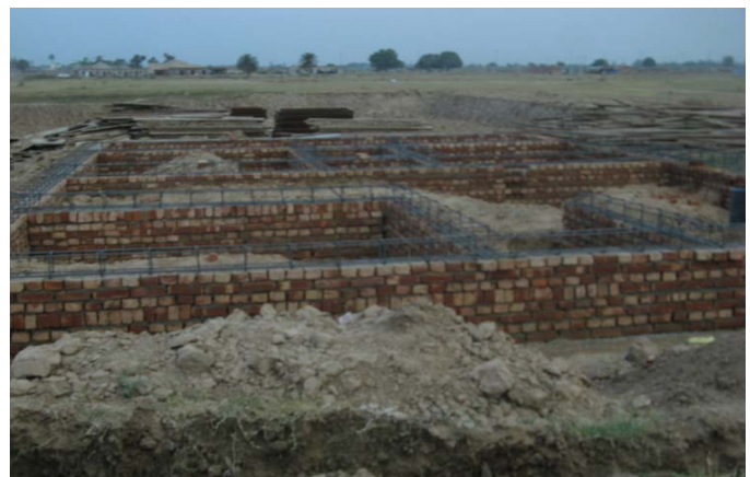
Construction in full swing on the plots handed over to the customers in Golf Links - I Mohali, Punjab
